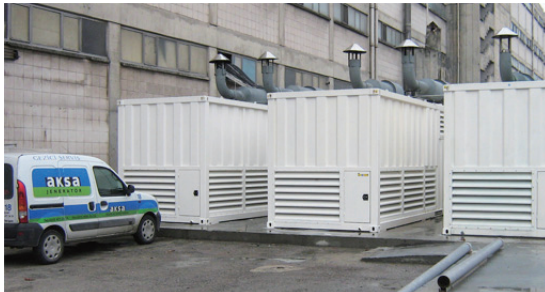
Moscow Ruihao PVC factory, 3 units 2250KVA, 400V container rites gensets runs weaver.
