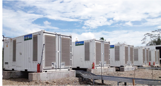
Philippines DMCI group, 18 units APD1513M-6 containerized gensets and parallel operation.
