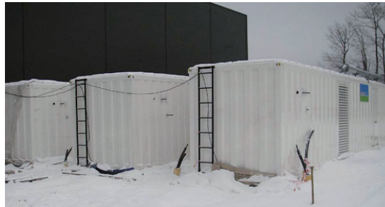
Moscow Ruihao PVC factory, 3 units 2250KVA, 400V container rites gensets runs weaver.
