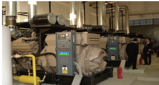
Istanbul international airport, 5 units 2000KVA, 6.3KV high voltage gensets runs weaver.
