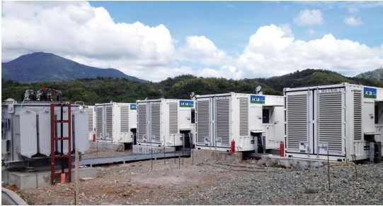
Philippines DMCI group, 18 units APD1513M-6 containerized gensets and parallel operation.
